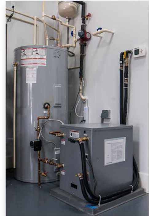
Dedicated Hot Water GHP (water-to-water GHP)
